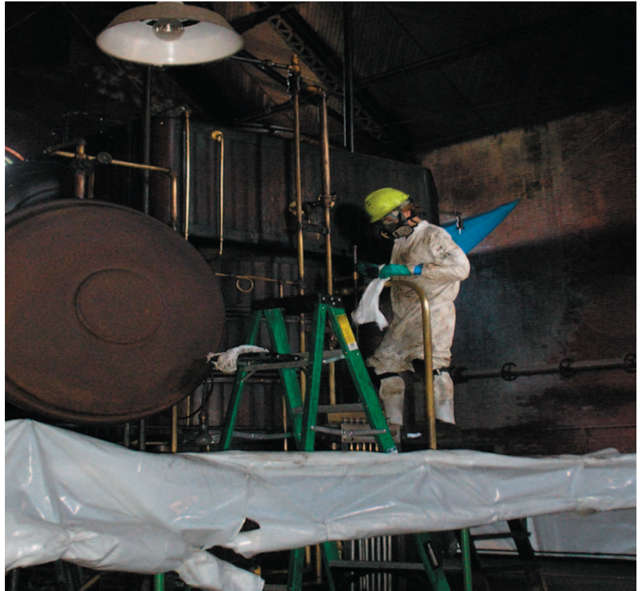
Restoration work underway at the Boston Waterworks
